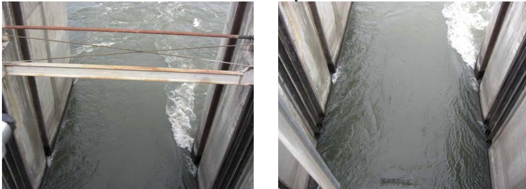
Photos 1 & 2 Water velocity before test conditions
